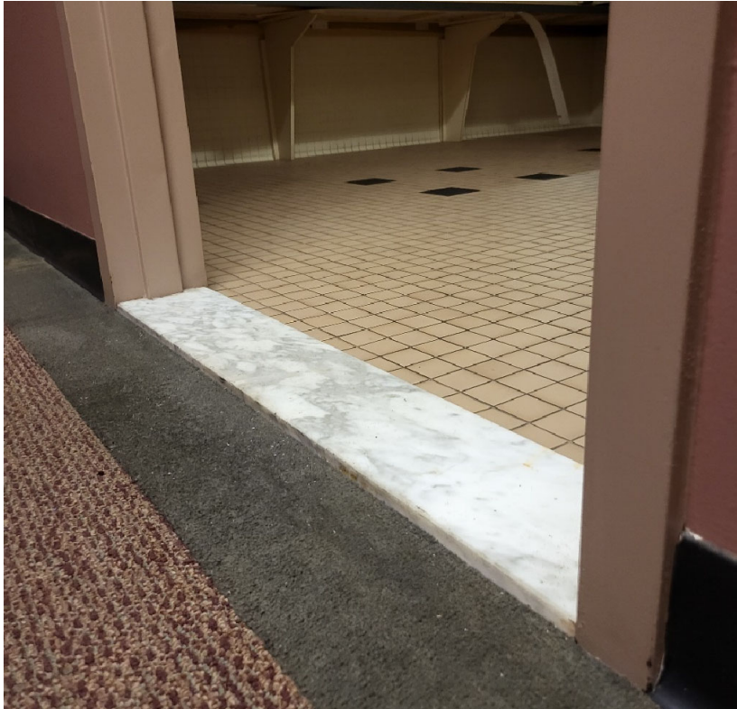
Existing Marble Threshold
