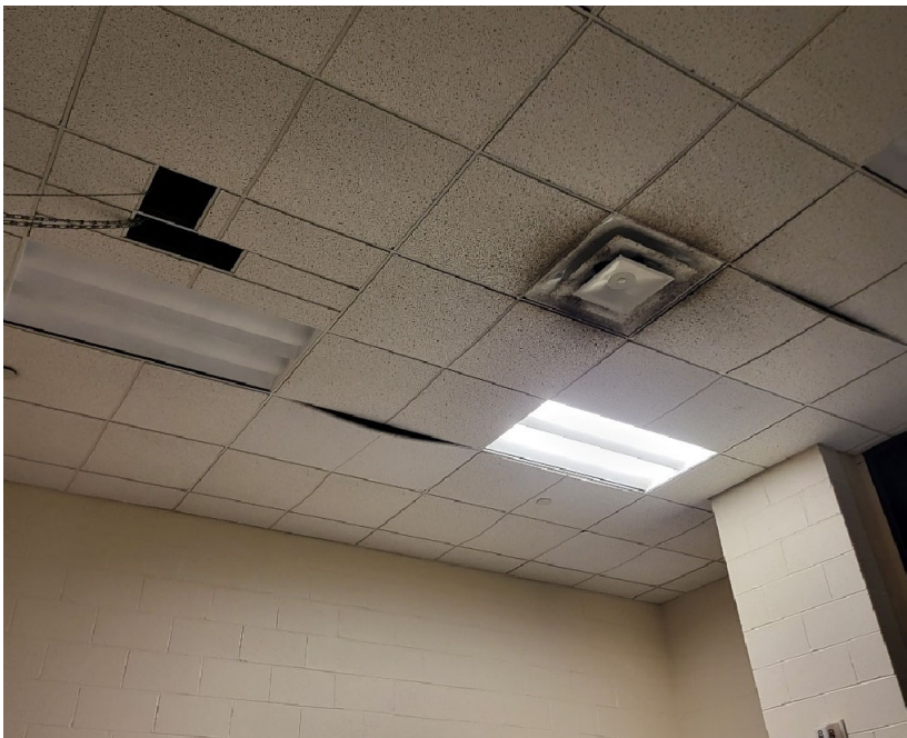
Existing Acoustical Ceiling Tile and Wall Finishes
